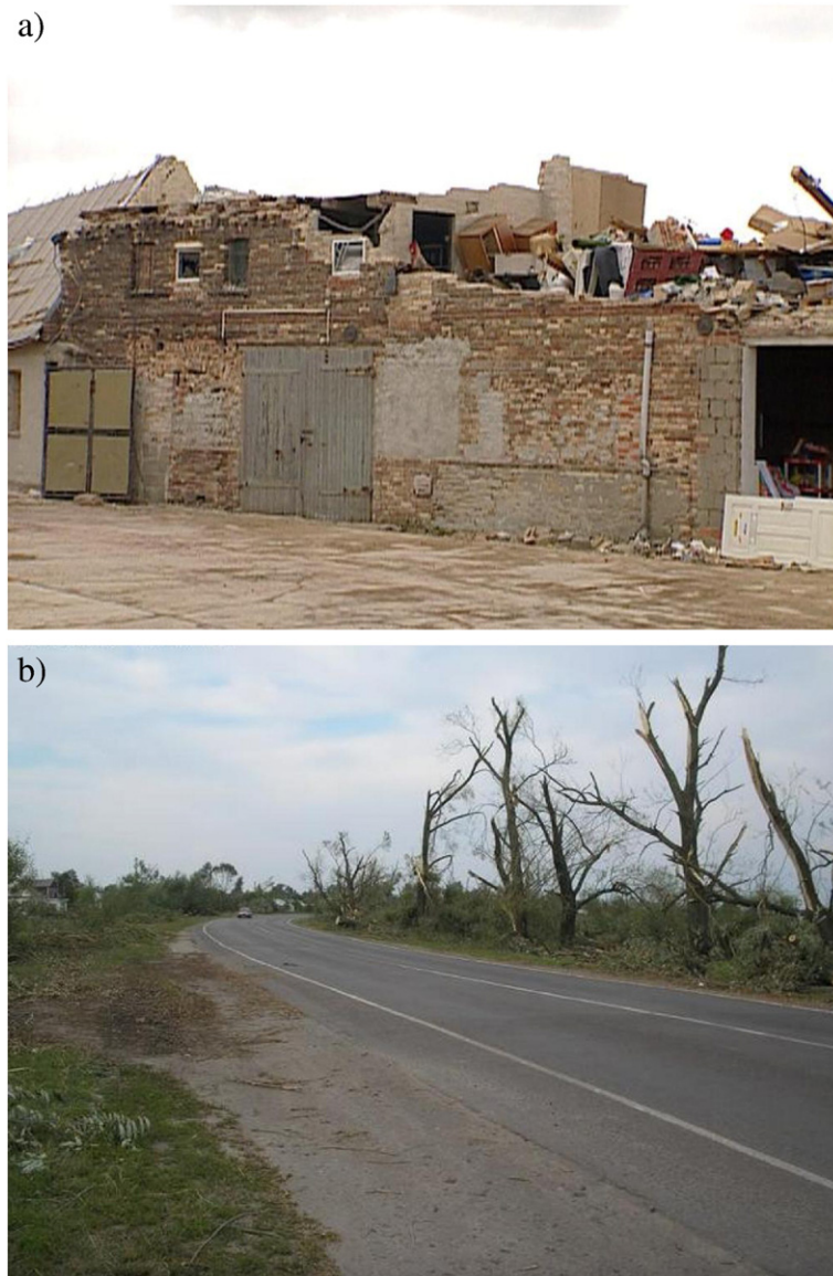
Fig. 13. T7 (F3+) damage. (a): Upper storey of outbuilding completely destroyed. Tornado, 23 June 2004, Micheln (Germany), Photo: Martin Hubrig. (b): Destroyed solitary trees with isolated debarking. Tornado, 22 July 2007, Turiysk (Ukraine), Photo: Olexandr Khilchuk.
