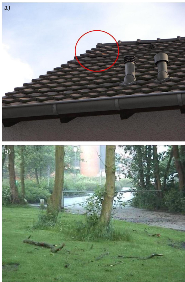
Fig. 6. T0 (F0–) damage. (a): Tiles slightly displaced. Downburst, 18 January 2007, Pulheim (Germany), Photo: Erik Dirksen. (b): Leaves, small twigs and dead branches snapped. Downburst, 4 June 2003, Schillig (Germany), Photo: Martin Hubrig.
