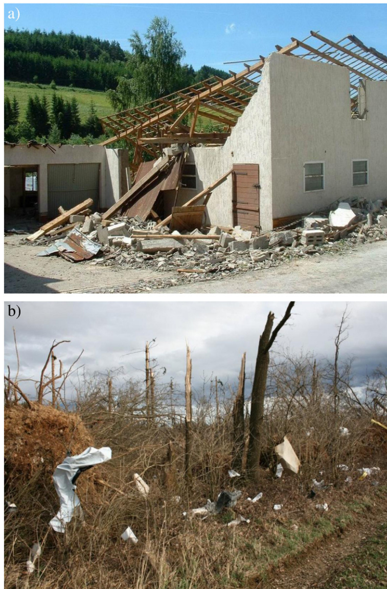
Fig. 12. T6 (F3–) damage. (a): Largely demolished and partly collapsed outbuilding. Tornado, 10 June 2003, Acht (Germany), Photo: Matthias Habel. (b): Completely destroyed sturdy but exposed forest edge. Downburst, 1 March 2008, Braunau am Inn (Austria), Photo: Alois M. Holzer.
