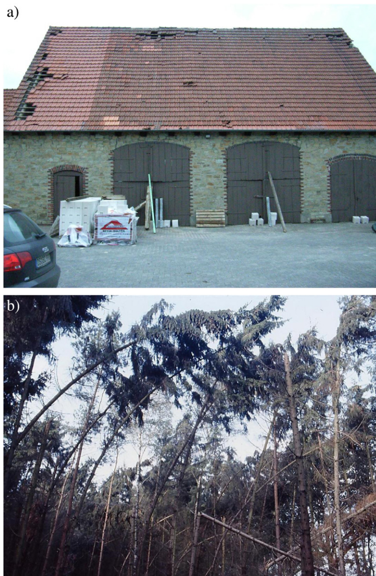
Fig. 8. T2 (F1–) damage. (a): Roof partially untiled. Downburst, 17 January 2007, Melle-Riemsloh (Germany), Photo: Martin Hubrig. (b): Permanently bent spruces. Downburst, 6 June 1998, Steinfurt (Germany), Photo: Martin Hubrig.
