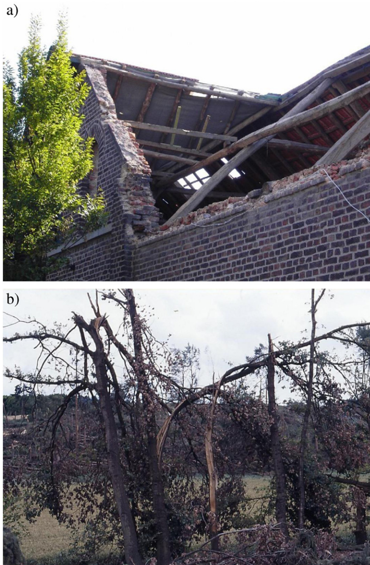
Fig. 11. T5 (F2+) damage. (a): Aged roof structure partly destroyed. Tornado, 18 July 2004, Tönisvorst (Germany), Photo: Thomas Sävert. (b): Heavily damaged edge trees. Tornado, 29 June 1997, Bissendorf (Germany), Photo: Martin Hubrig.
