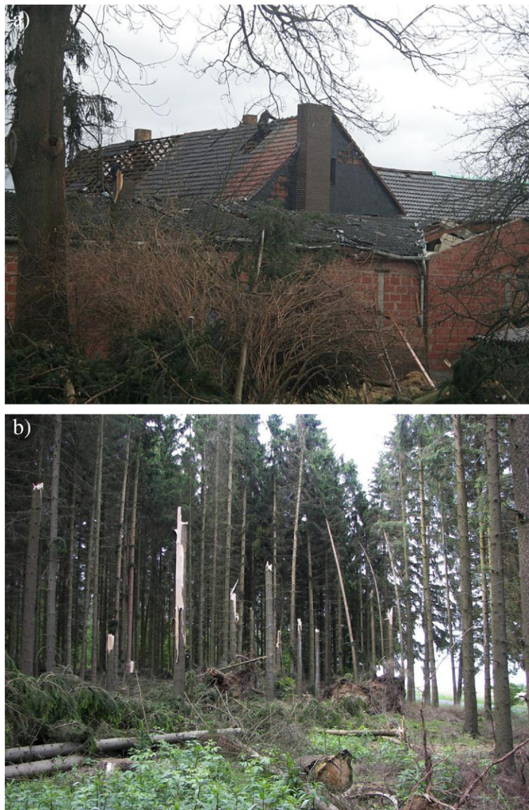
Fig. 9. T3 (F1+) damage. (a): Roof largely untiled. Tornado, 1 March 2008, Uttershausen (Germany), Photo: Eyk Neidert. (b): Spruce forest with bending and snapping; edge intact. Tornado, 29 May 2007, Borler (Germany), Photo: Erik Dirksen.
