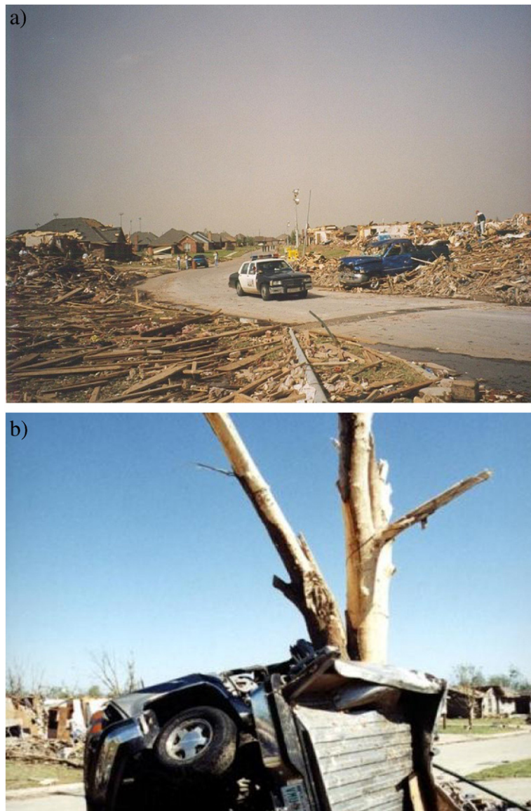
Fig. 16. T10/11 (F5) damage. (a): Complete destruction (total loss) of buildings. Tornado, 3 May 1999, Moore, OK (USA), Photo: Mike Branick, NWSFO. (b): Widely debarked tree and destroyed pickup truck. Tornado, 3 May 1999, Moore, OK (USA), Photo: Kevin Kelleher.
