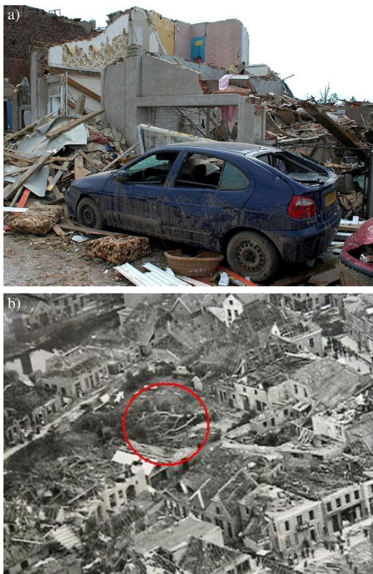
Fig. 15. T9 (F4+) damage. (a): Massive (brick) house ruined down to base walls. Tornado, 3 August 2008, Hautmont (France), Photo: Bjoern Stumpf. (b): Largely debarked Tree. Tornado, 10 August 1925, Borculo (Netherlands), Photo: Stormrampmuseum Borculo.
