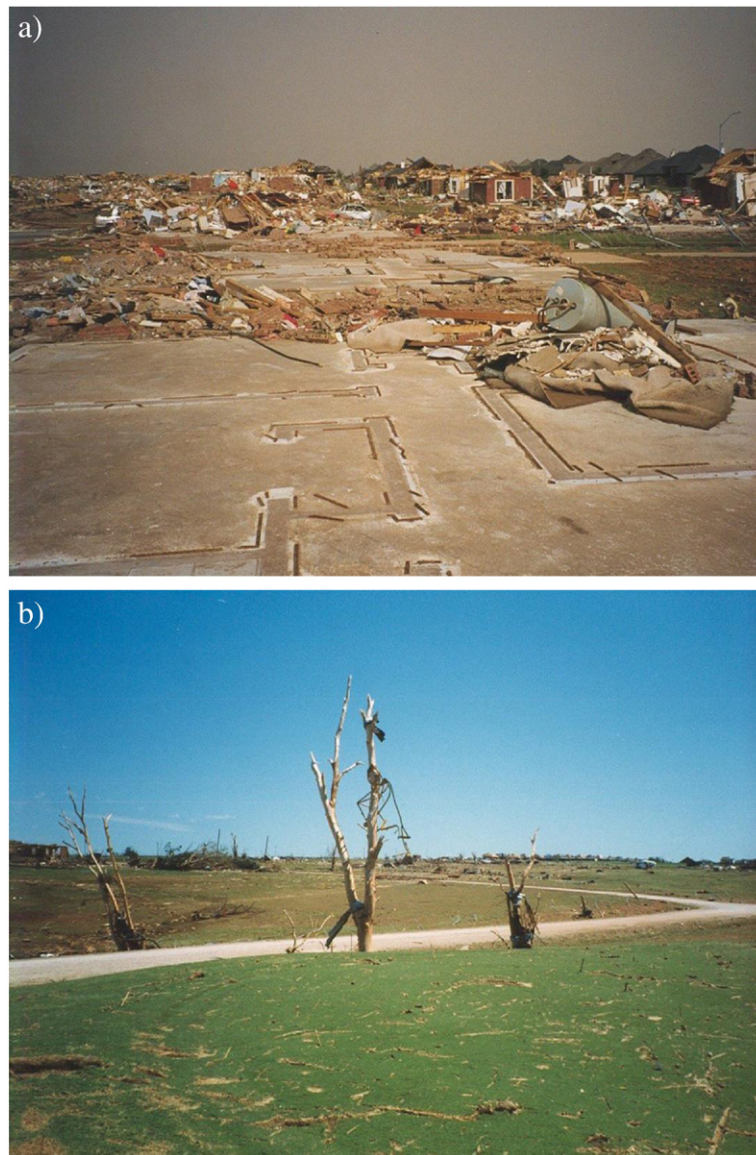
Fig. 17. T10/11 (F5) damage. (a): Buildings blown away from foundation. Both panels tornado, 3 May 1999, Moore, OK (USA), Photos: Mike Branick, NWSFO. (b): Completely debarked solitaire tree ruins.
